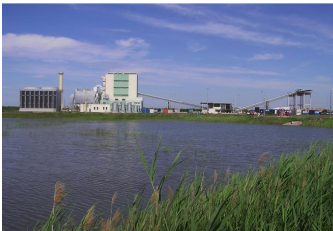
20 MW biomass plant, Hungary
